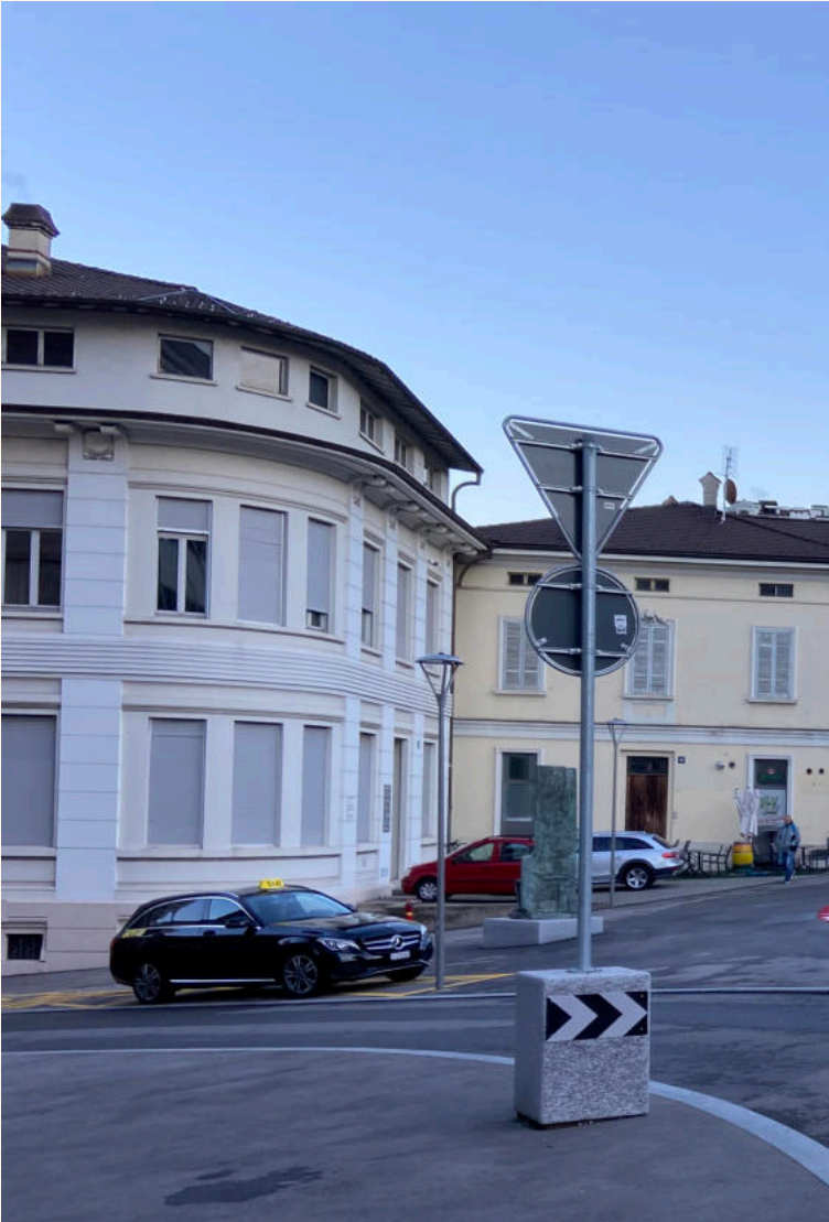
FFS TRAIN STATION, CHIASSO (CH)
